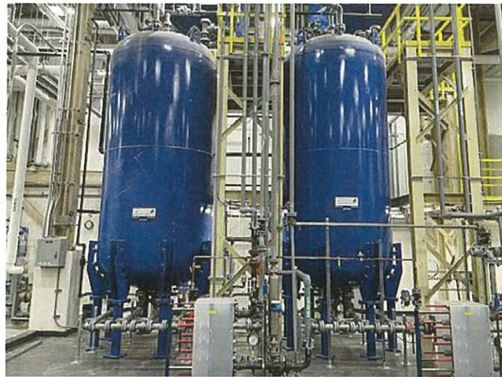
Glass-lined sulfonation tanks weighing over 30,000 pounds each help ResinTech turn virgin polymer into the company's newest flagship product — non-solvent, sodium form cation resin. ©ResinTech, Inc. All rights reserved.
